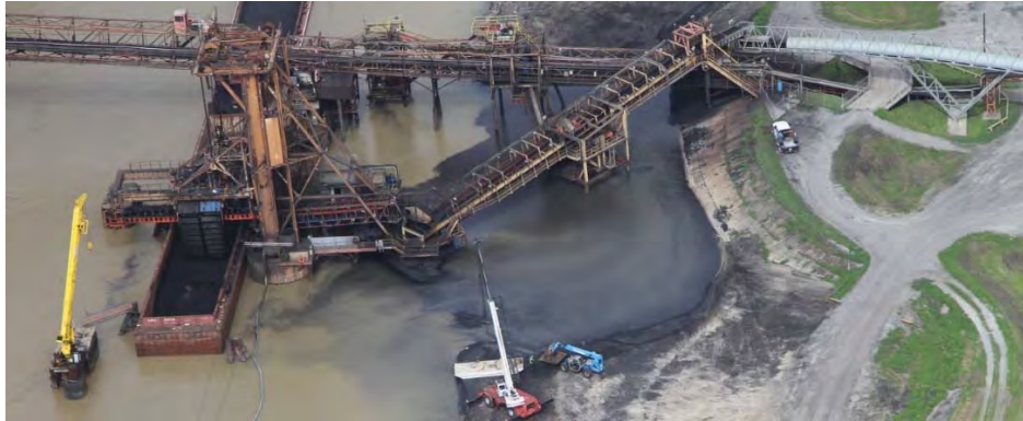
Discharges to the Mississippi River from the United Bulk coal terminal in Plaquemines Parish
